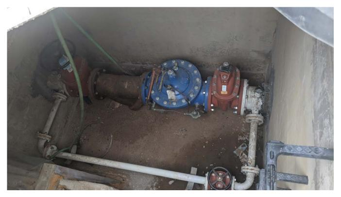
Attachment: 3 Severity: Significant Facility ID: 043 Category: F310 Attachment Comments: Since tank 043 is abandoned, the supplier must disconnect it from distribution by more than just a valve. The picture shows the abandoned tank and the valve isolating it from distribution currently.
